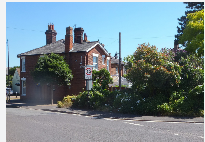
Figure 102: Local positive example of corner treatment where the building façades overlook the street on both sides, whilst hedges and trees create a curved boundary around the plot offering good visibility for pedestrians, Foundry Lane.
