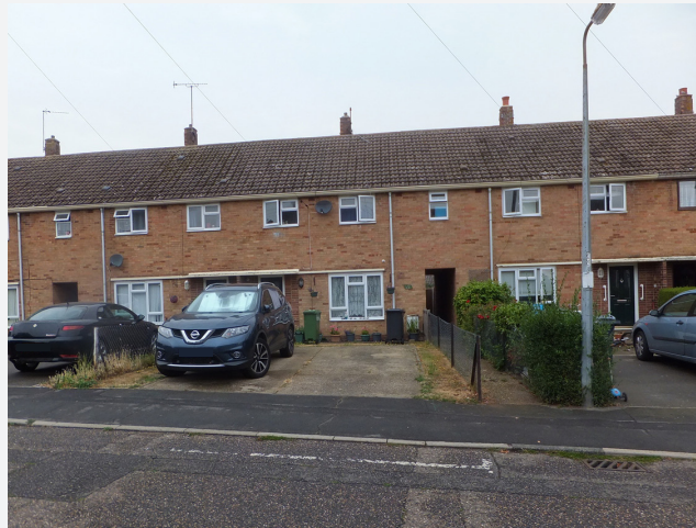
Figure 98: The building massing along Atlas Road in the Mixed Residential areas is consistent with subtle variations.
