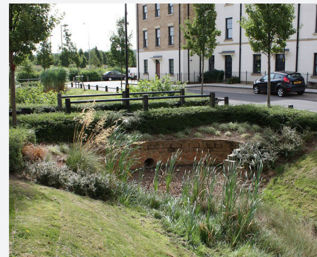
Figure 73: Example of swales check dam integrated with a crossing point, somewhere in UK.
