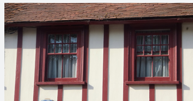
Casement windows with painted timber frame
