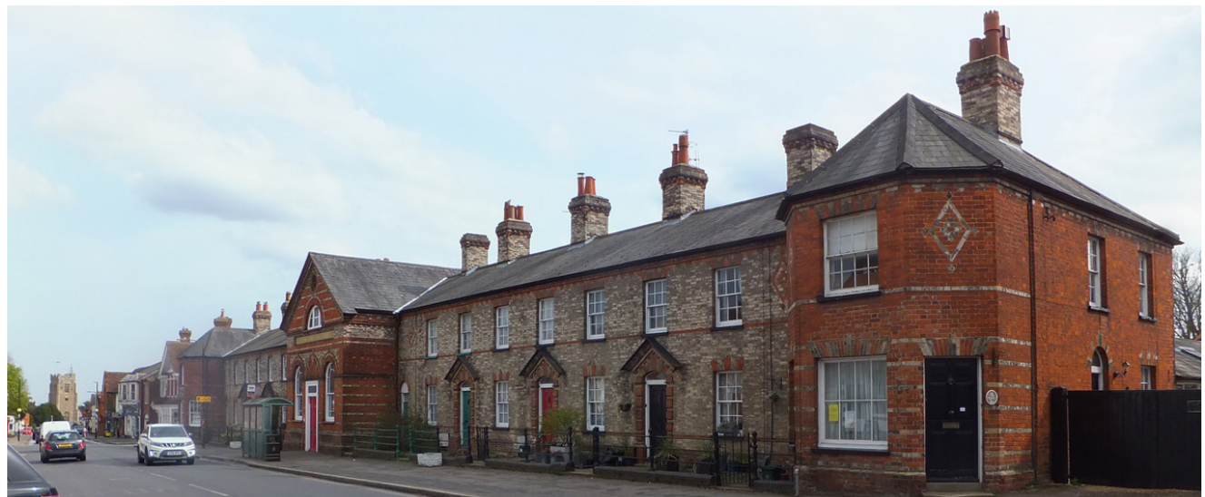
Figure 16: Rows of terrace houses on narrow plots providing continuous frontages along the High Street, comprising of residential houses, shops and civic uses such as the public library.
