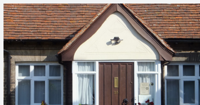
Gabled porch with timber door
