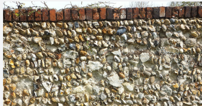
Local stone combined with brick
