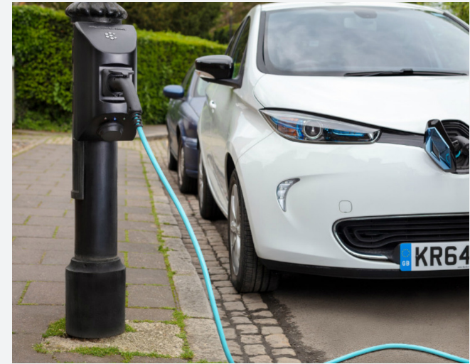
Figure 63: Example of on-street electric vehicle charging points.
