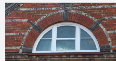
Bow window on listed building
