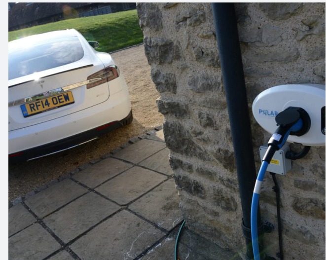
Figure 65: Example of off-street electric vehicle charging points.
