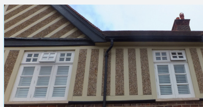
Modern casement windows
