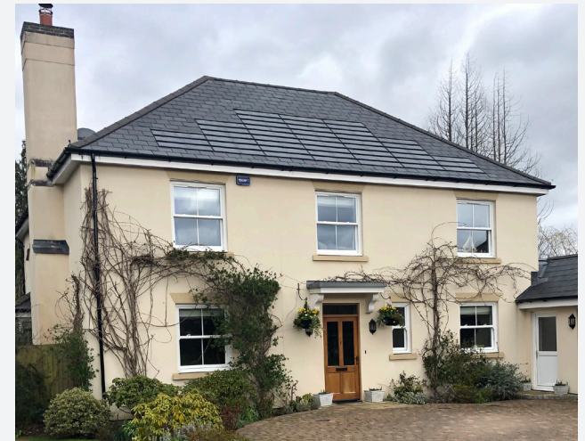
Figure 108: Use of shingle-like solar panels on a slate roof, with the design and colour of the solar panels matching those of the adjacent slate tiles.
