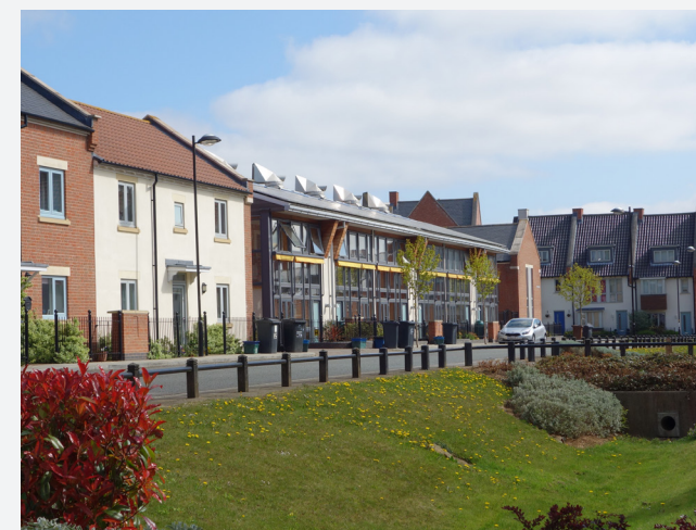
Figure 70: An example of a SuDS corridor - Upton Urban Extension, Northampton.
