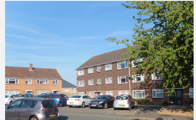
Figure 88: Flats on De Vere Road with green verges and parking court at front.
