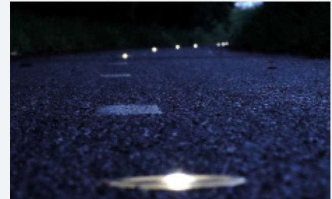
Figure 106: Example of a foot/cycle path which is lit by solar cat's-eye providing some light for pedestrian and cyclists without creating any disturbance to the nearby properties or unacceptable levels of light pollution.
